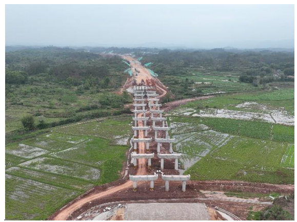
傍江下大桥现状 (2023.4)
